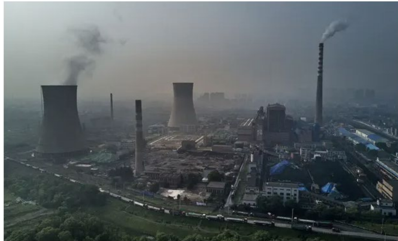
📷 A state-owned coal-fired power plant in Huainan, Anhui province, China. Photograph: Kevin Frayer/Getty Images
